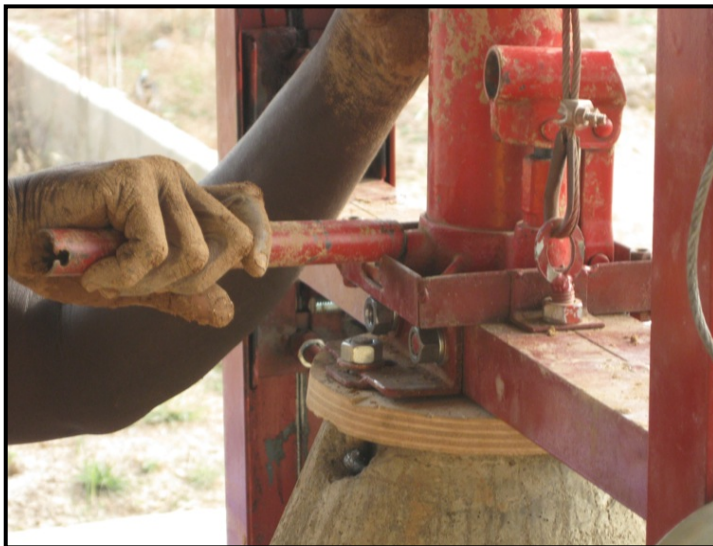
Figure 4-9: Affixing the lever to the jack
